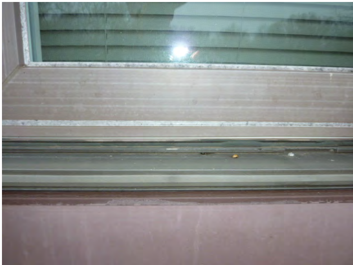
Original 1976 windows typically have failing gaskets and other age-related wear/deterioration.
