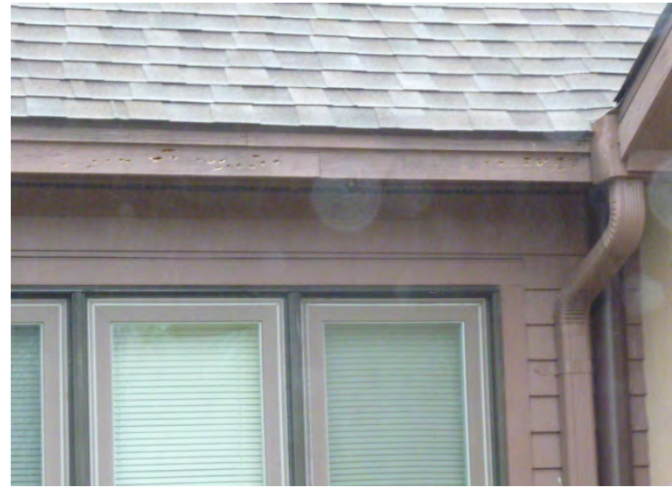
Original 1976 wood trim was not replaced as part of 2008 exterior renovation scope of work.
