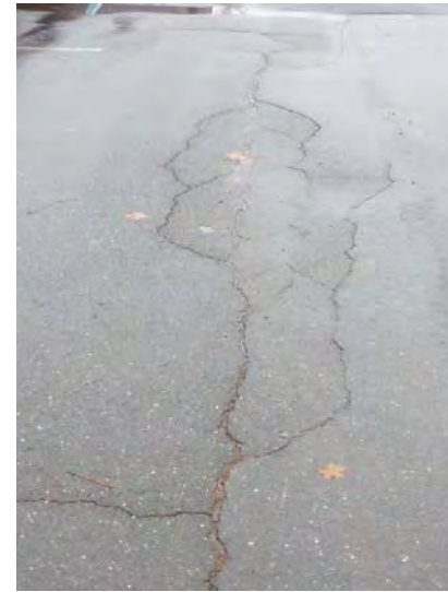
Sealcoat and striping of asphalt drive and parking is needed in the near-term
